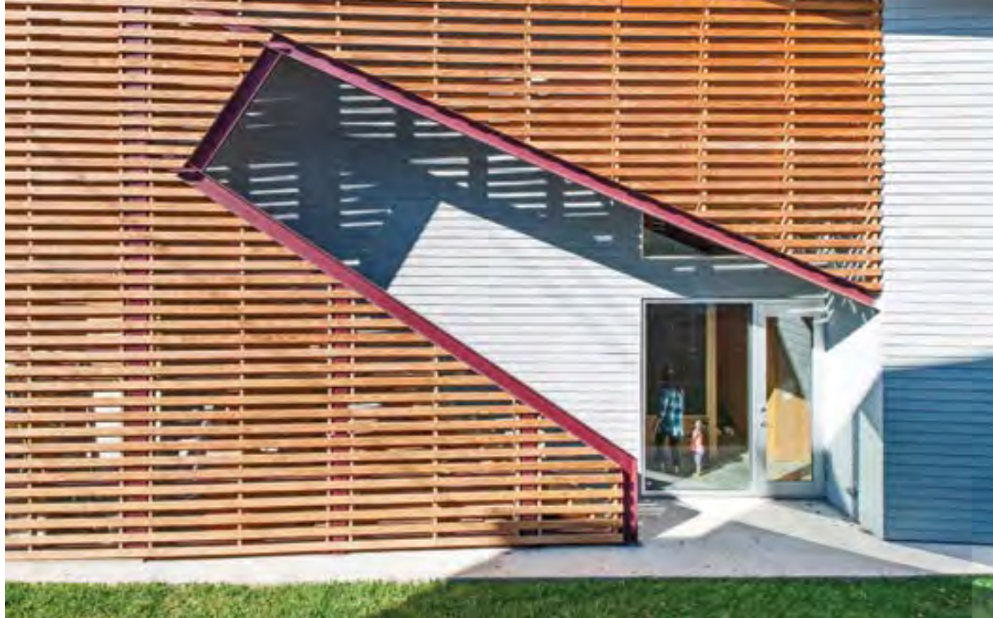
An exterior staircase provides a separate entrance for second floor inhabitants and direct access to the front porch. The wooden slats provide privacy, but also let in sunlight and air to help ventilate the home.
